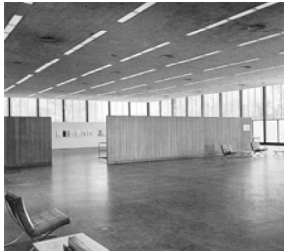
Image 31. – IIT Crown Hall interior view
